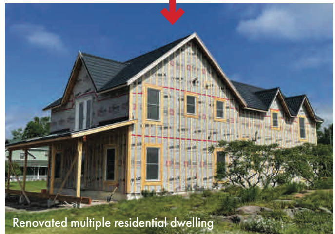
Example of a thoughtful renovation on Channel Street.
