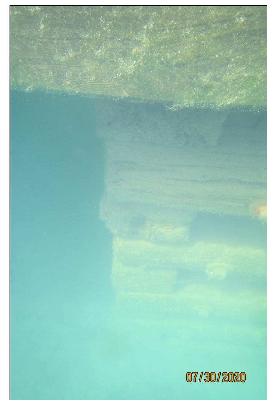
Underside of South Dock on East Side
