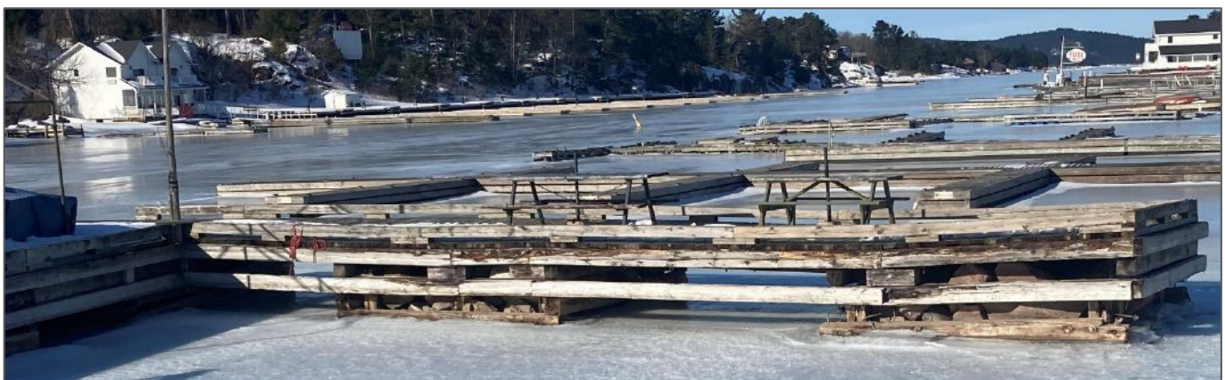
Figure 18: Killarney Wharf Finger Dock
