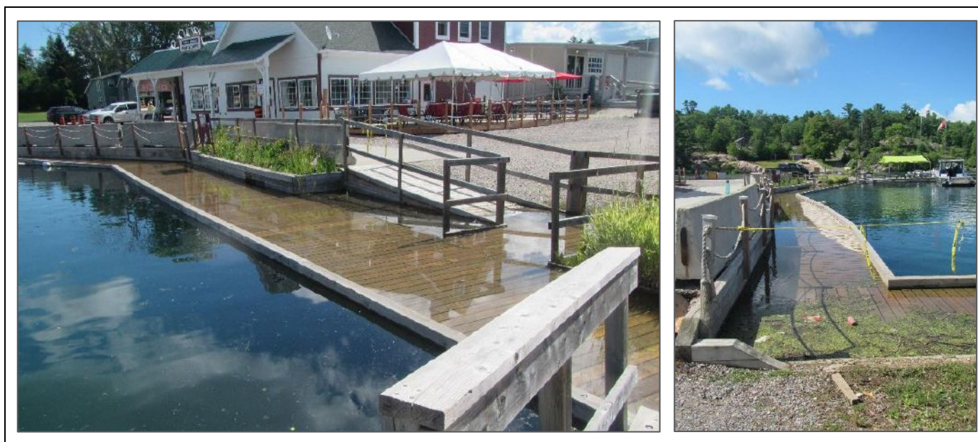
Figure 6: Flooding at the Killarney Municipal Wharf (July 2020)
