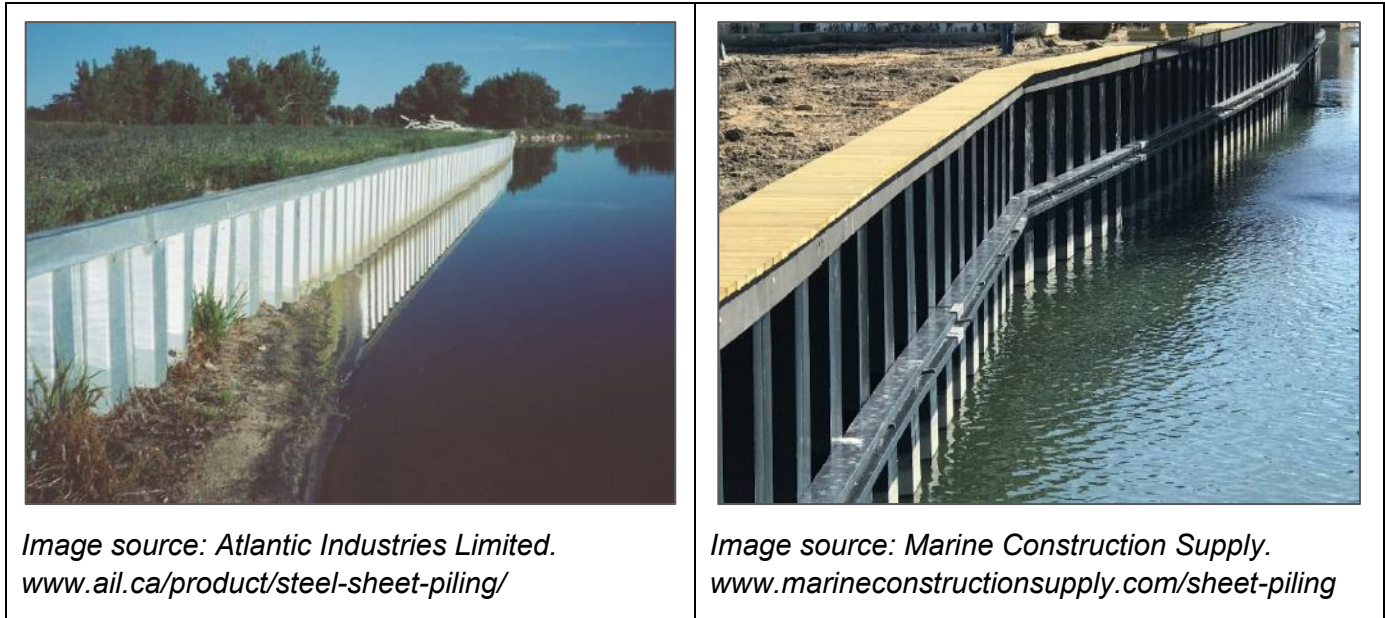
Figure 17: Examples of Sheet Pile Walls
