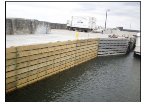
Example of timber fender
