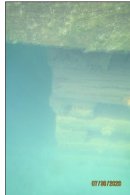
Underside of South Dock on East Side
