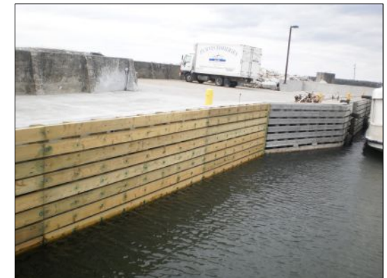
Example of timber fender
