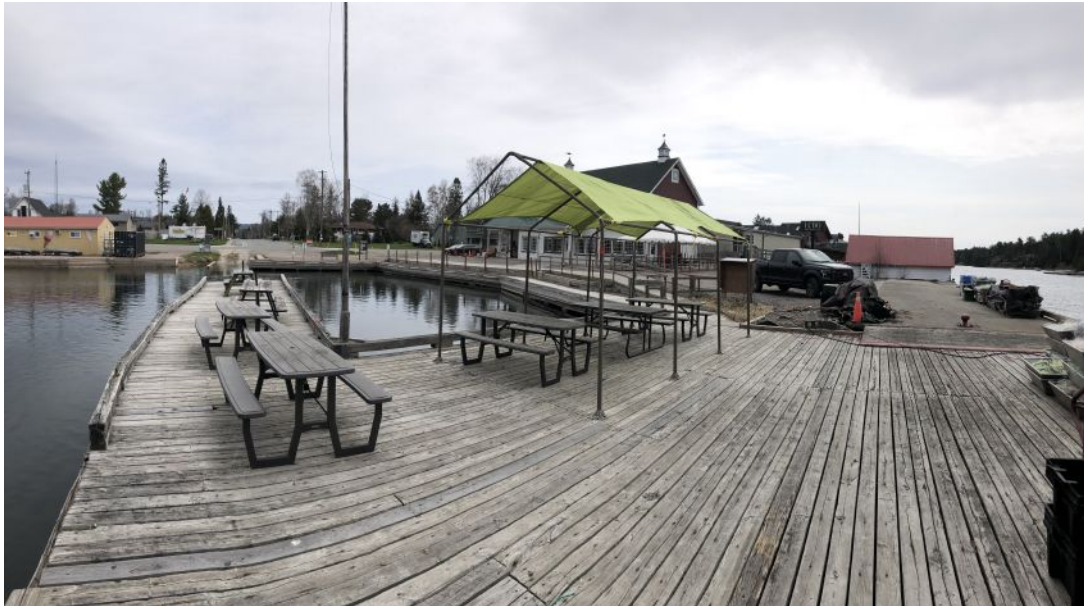
Figure 14: Overview from Southwest Corner (looking northeast)
