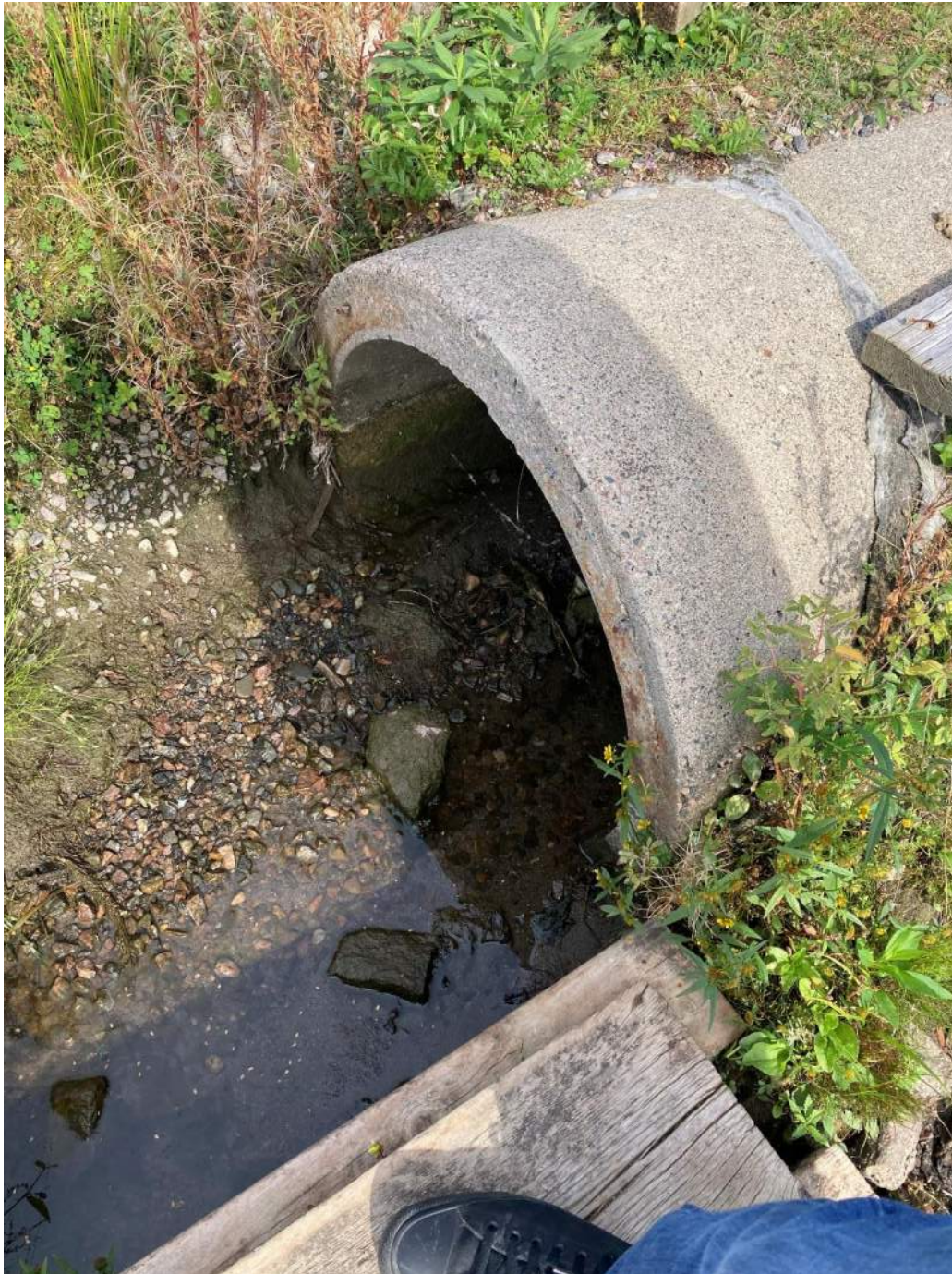
Photograph No. 17 Storm sewer discharge to Killarney Channel in northwest area of the Site.
