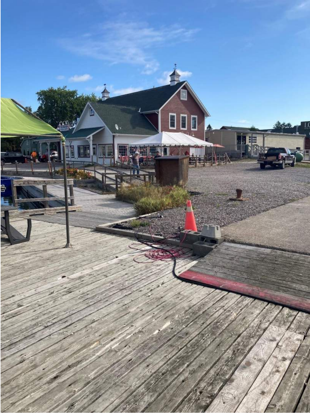
Photograph No. 1 View of the Site from the SW corner (looking NE).
