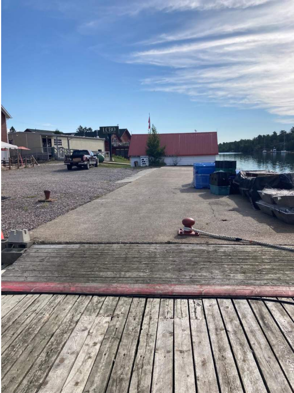
Photograph No. 2 Property line along south side of the Site (Killarney Channel along right side of image).
