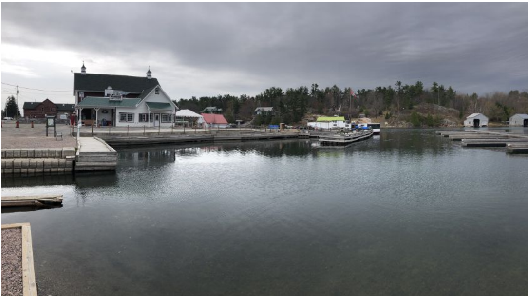
Figure 15: Overview from Northwest Corner (looking southeast)
