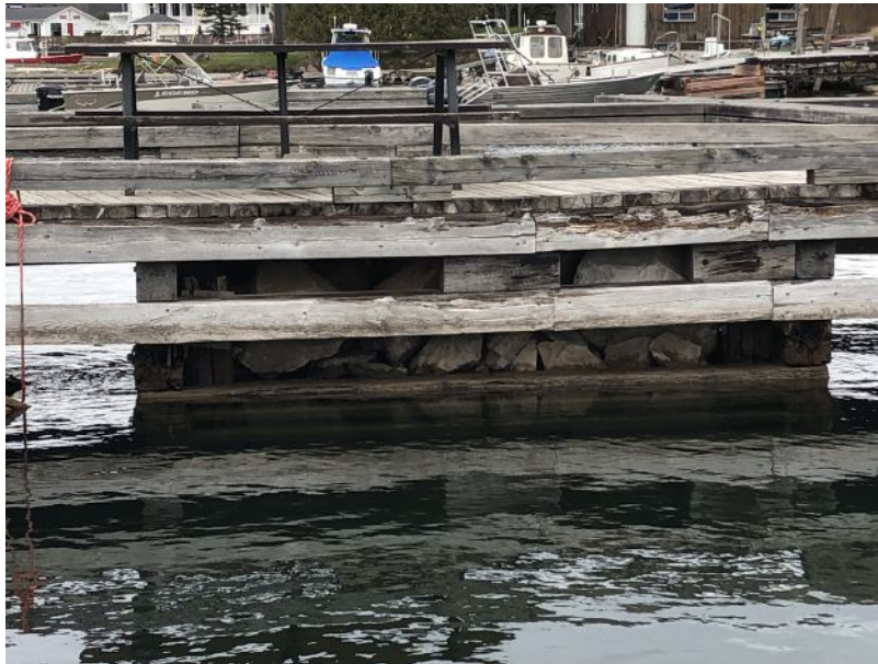
Figure 16: Typical Rock Filled Crib
