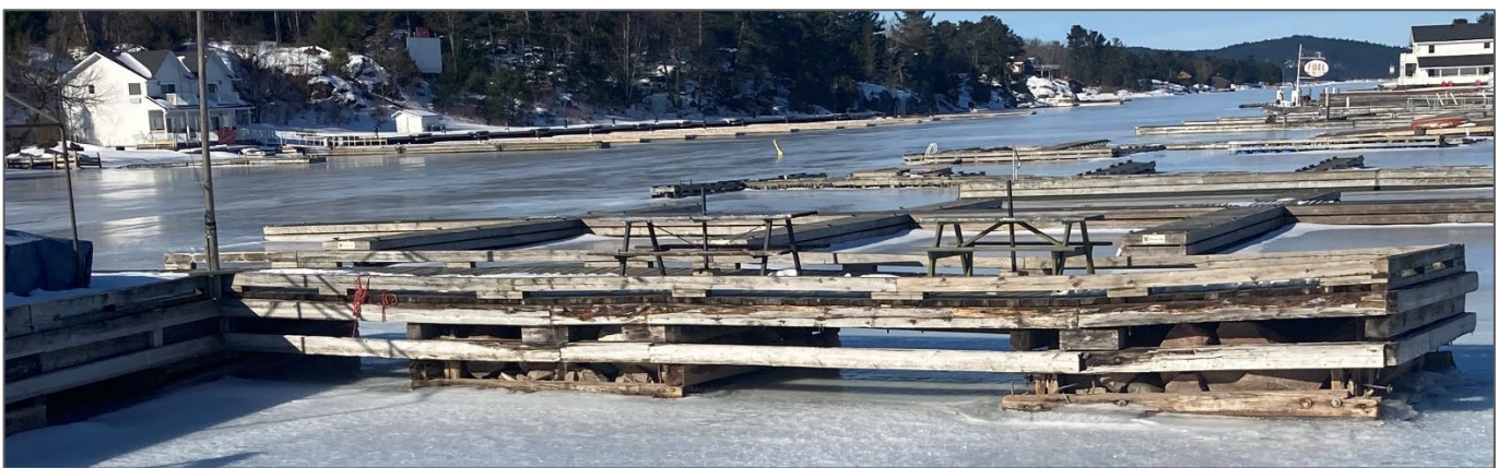
Figure 18: Killarney Wharf Finger Dock
