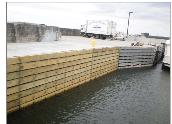
Example of timber fender
