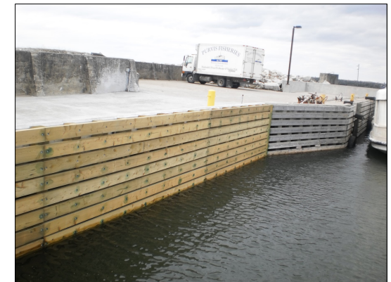
Example of timber fender
