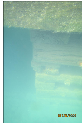
Underside of South Dock on East Side
