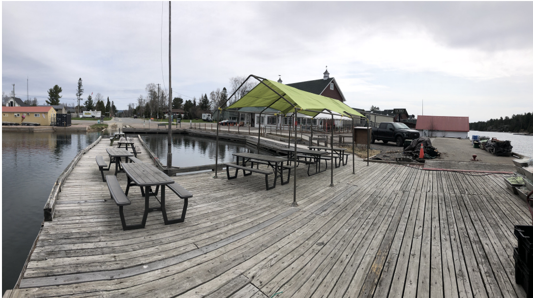
Figure 14: Overview from Southwest Corner (looking northeast)
