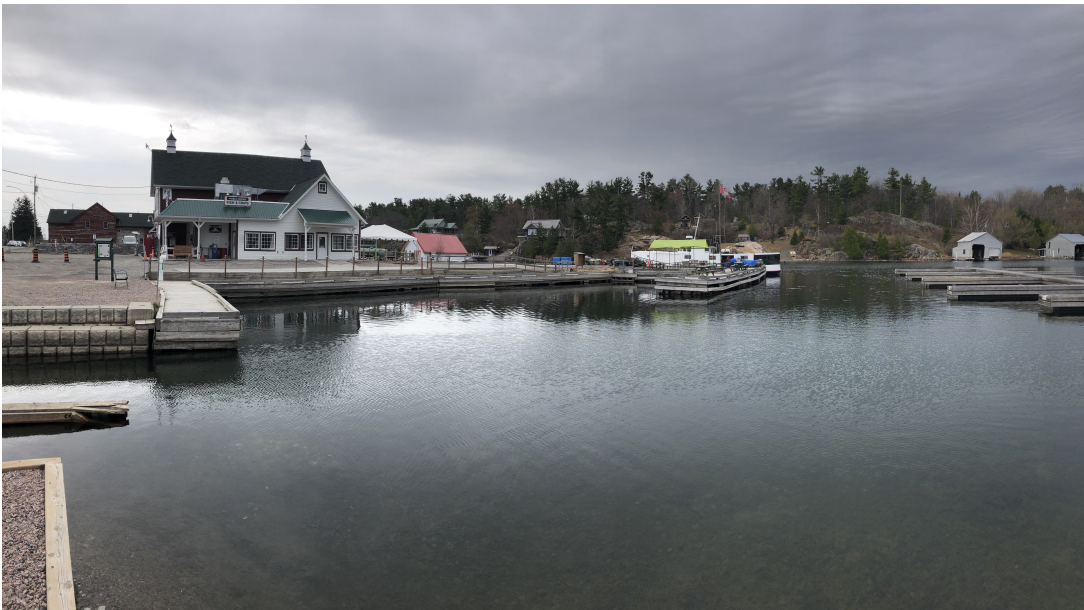
Figure 15: Overview from Northwest Corner (looking southeast)
