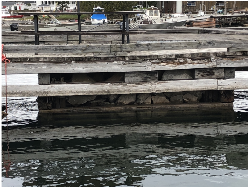
Figure 16: Typical Rock Filled Crib
