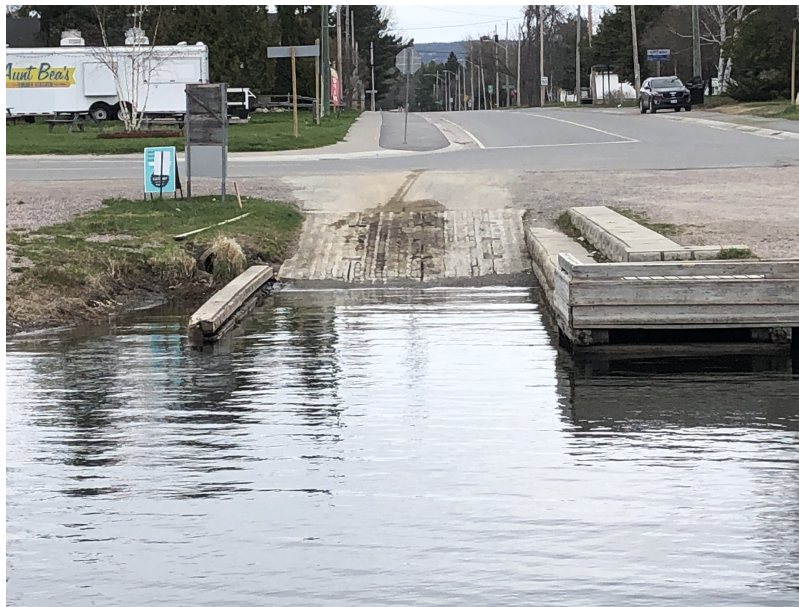
Figure 7: Existing Boat Launch and West End of North Section (looking north)
