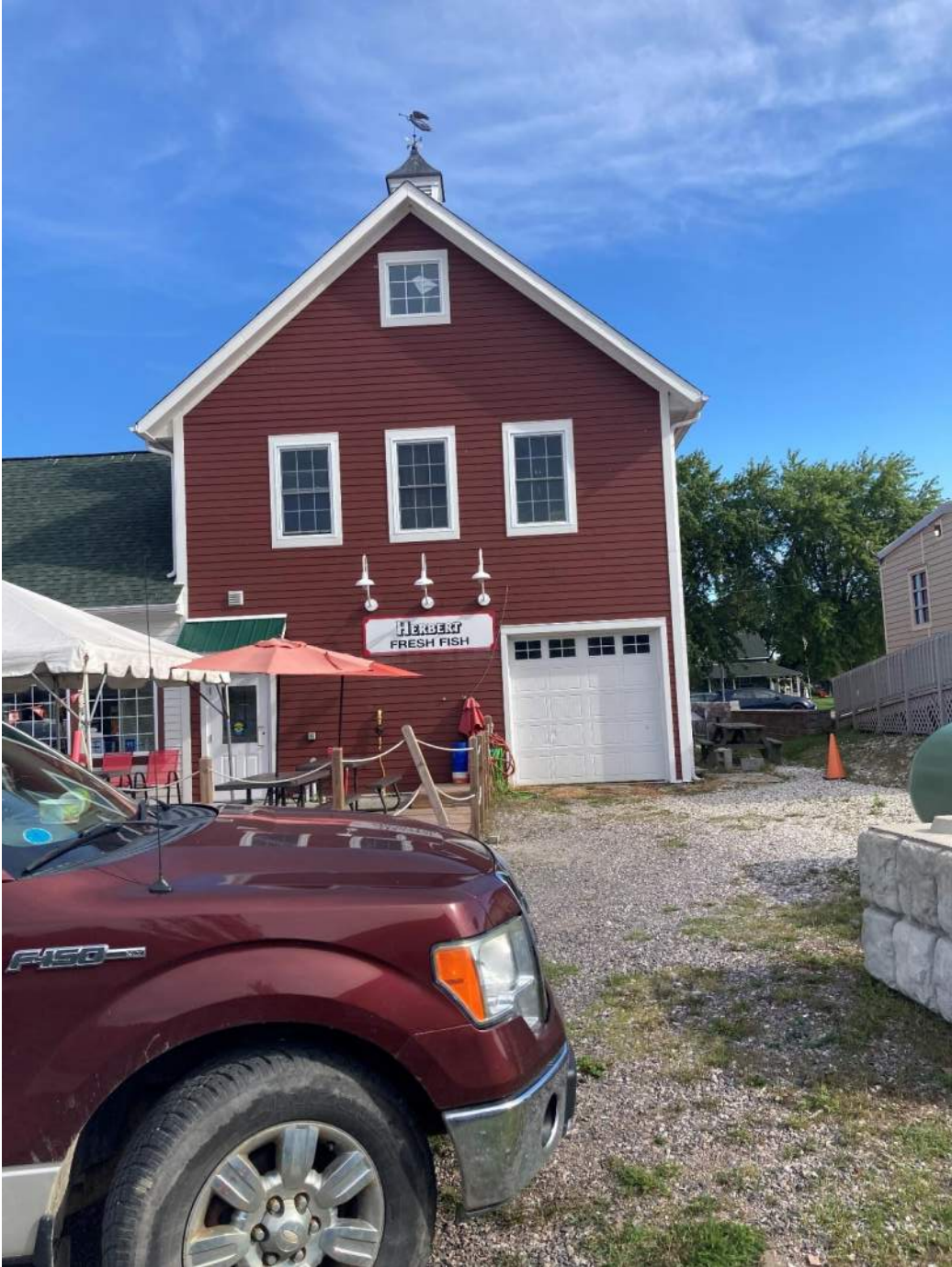
Photograph No. 7 – South side of central building.
