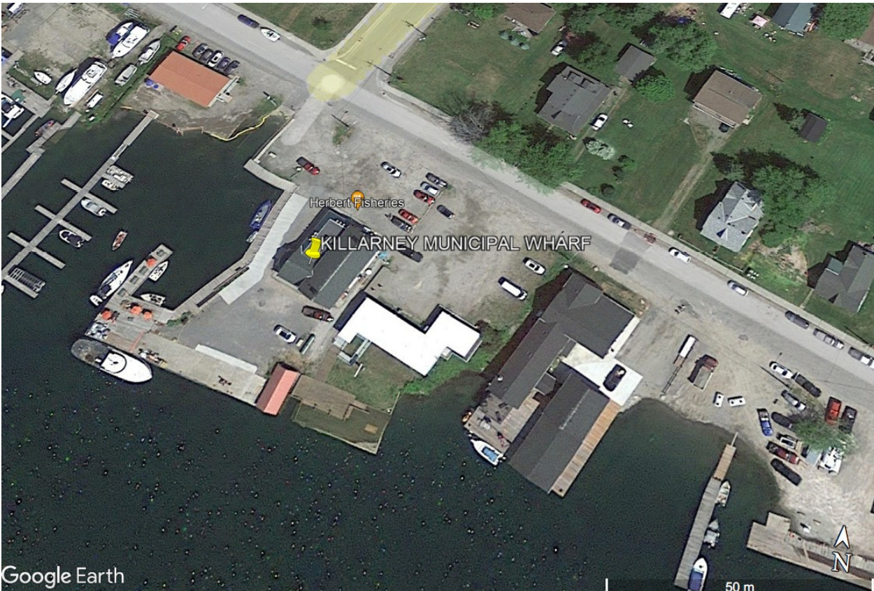
Figure 2: Existing Killarney Municipal Wharf
