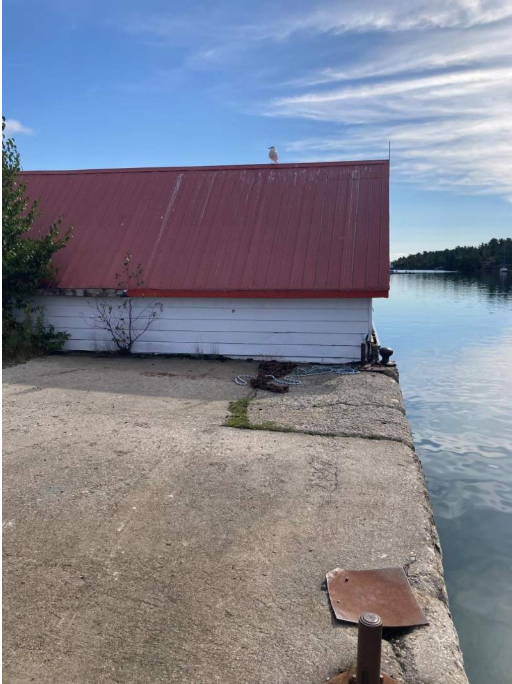
Photograph No. 3 Storage shed along south border of the Site.
