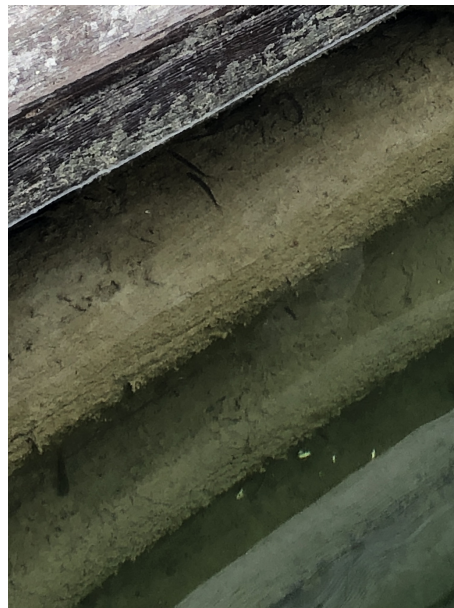
Figure 17: Typical Rock Filled Crib Below Water Line
