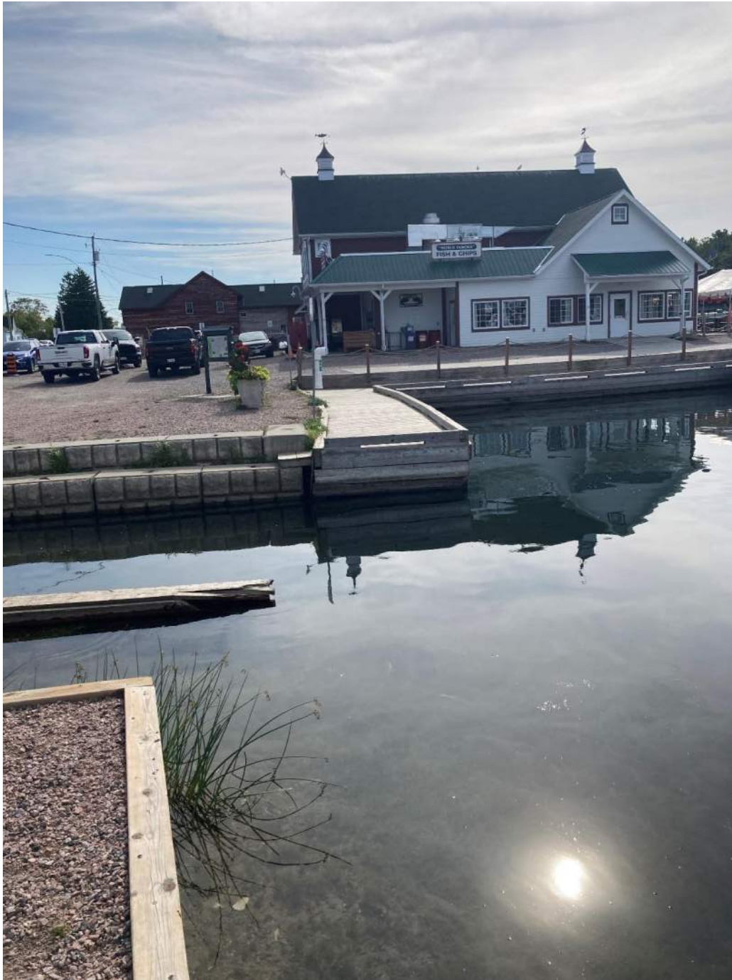
Photograph No. 21 Natural ground (left of retaining wall) and engineered ground (right of retaining wall) boundary.
