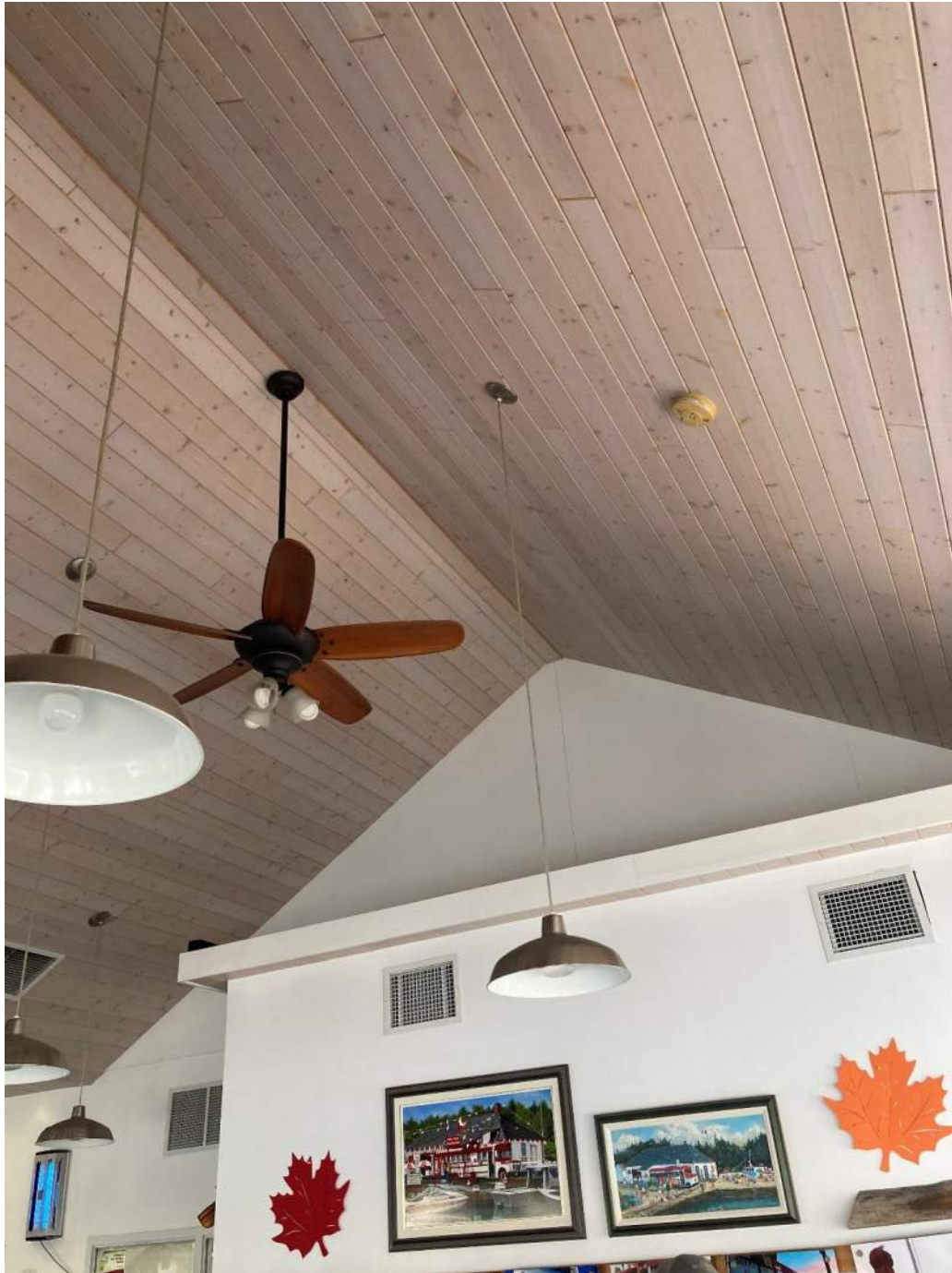
Photograph No. 15 Interior walls and ceiling materials of central building. Outside walls consisted of siding.
