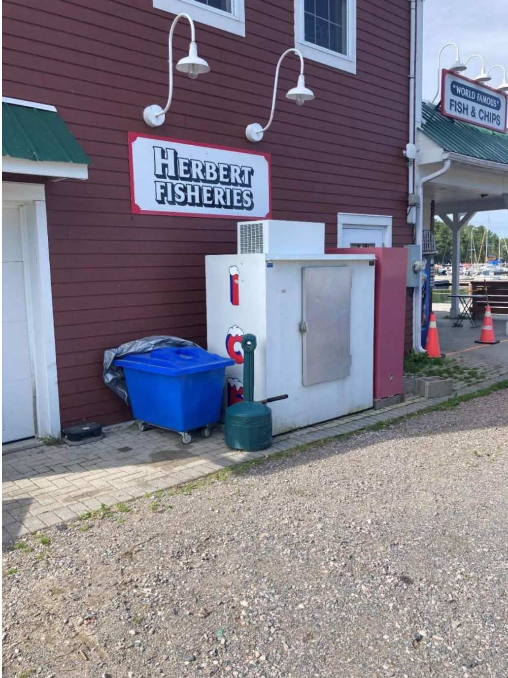
Photograph No. 23 Retail freezer unit on north side of central building (good condition).
