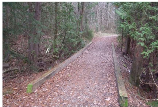
Photo 4 : Curb at Embankment
